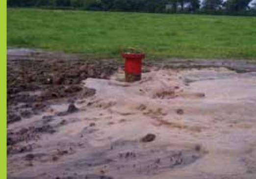
1. Brine flowing from the area surrounding the red wellhead casing
