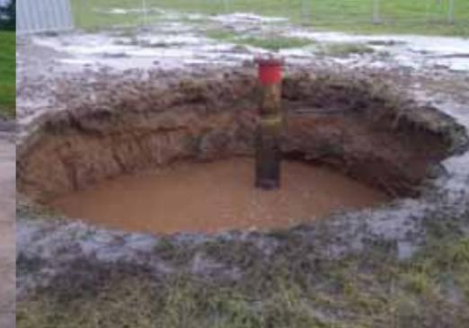
2. The air and brine flow eroded the soil surrounding the casing causing a hole to develop which filled with brine
